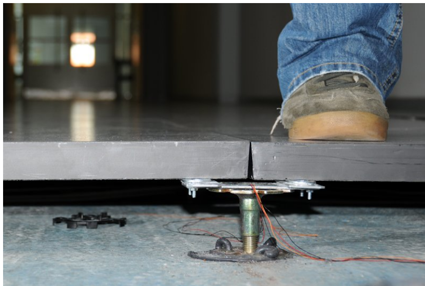
(b) Floor tiles rest on columns.
